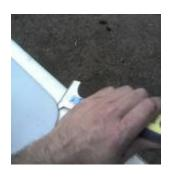
Repair 3 Using a paint scraper to start prying off the deck.
